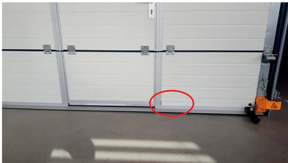
SD01/1 – po instalaci
