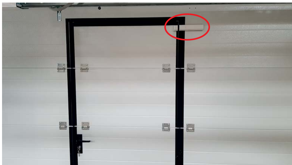
SD01/2 – po instalaci
